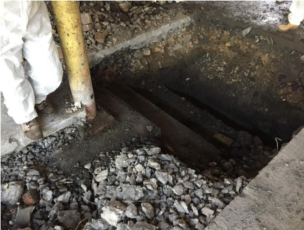
Photo 31: Tiered spread footing
