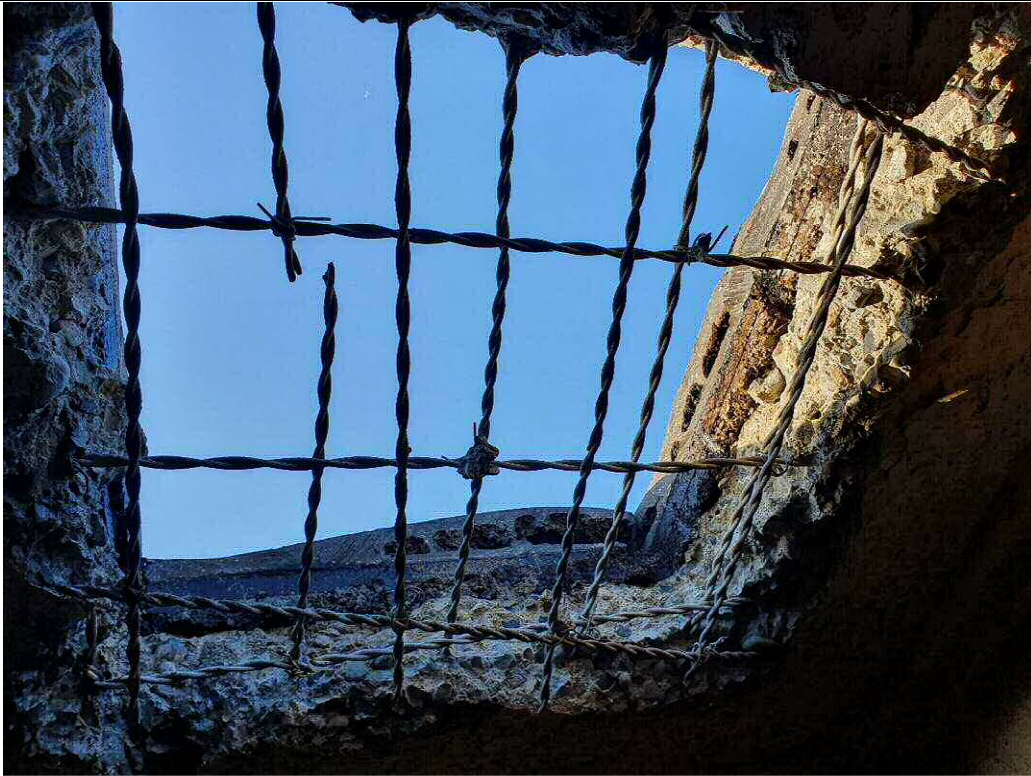
Roof Slab Reinforcing
