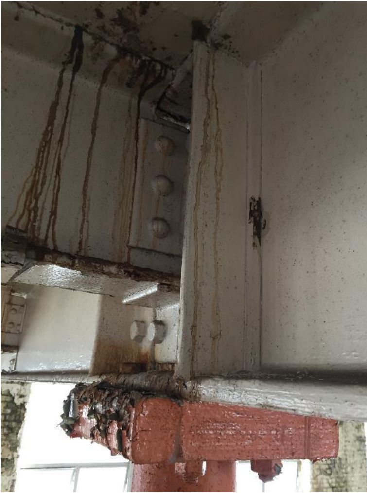
Photo 12: Typical column head connection
