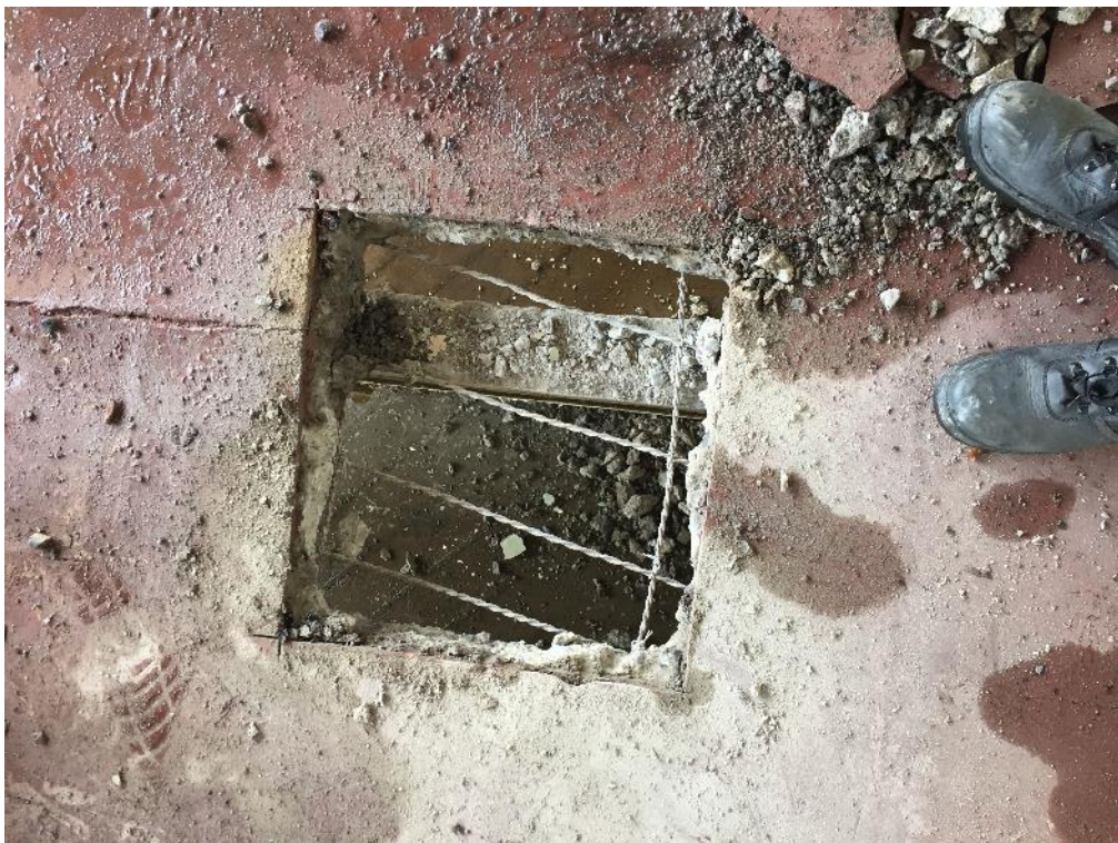
Photo 27: Level 3 reinforcement
