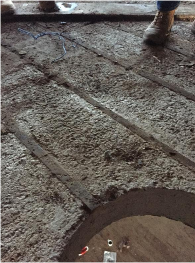
Photo 23: Core sample, with non-structural screed with timber batons
