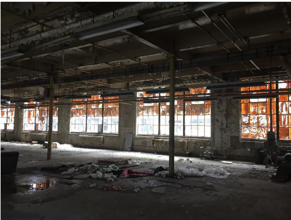
Photo 2: Original Building Condition
