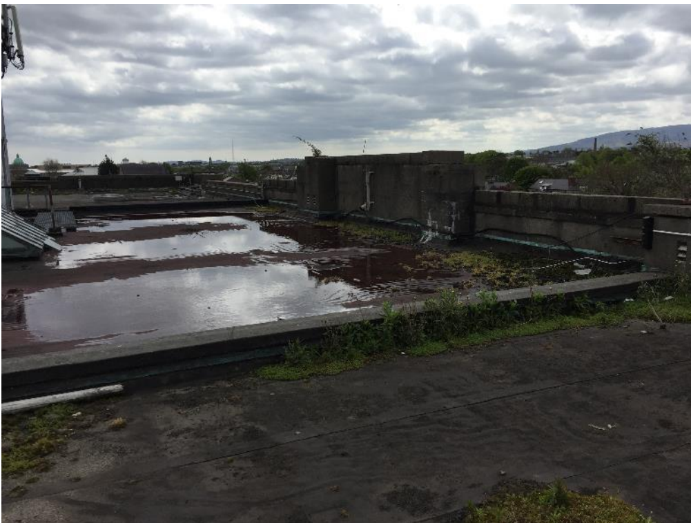
Photo 9: Original Building Condition
