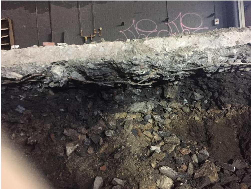
Photo 21: Ground Floor Slab
