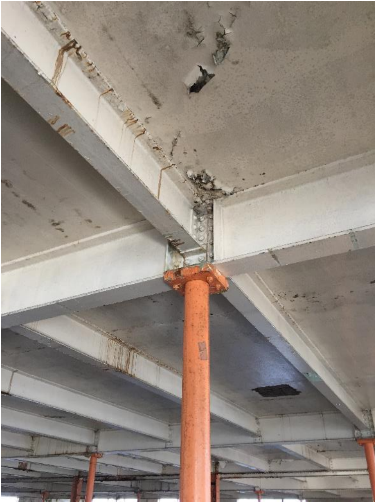
Photo 11: Typical Ground/First Column and beam
