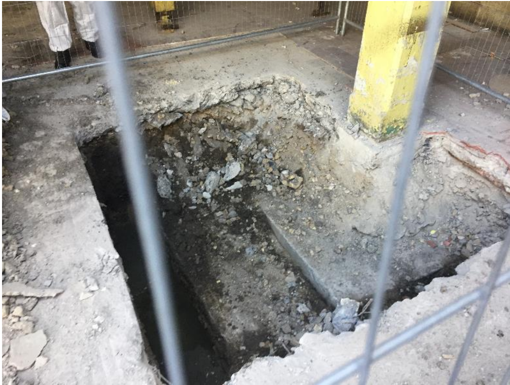
Photo 29: Tiered spread footing
