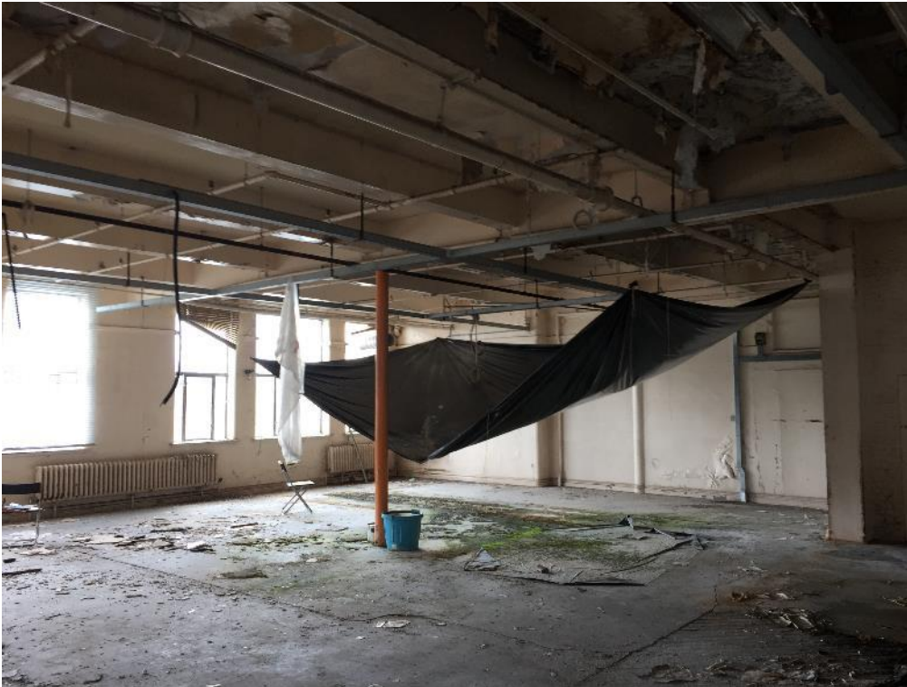
Photo 5: Original Building Condition
