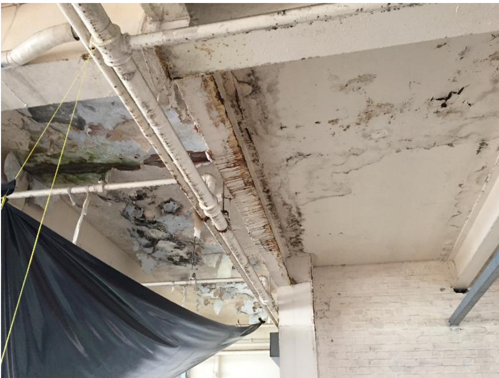
Photo 6: Original Building Condition
