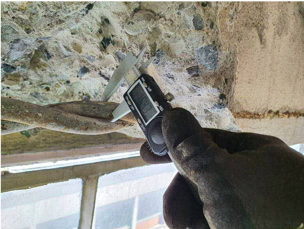
Beam above windows reinforcing steel
