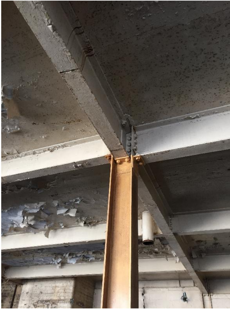
Photo 13: Level 2 column (1930's section) with level 3 beams
