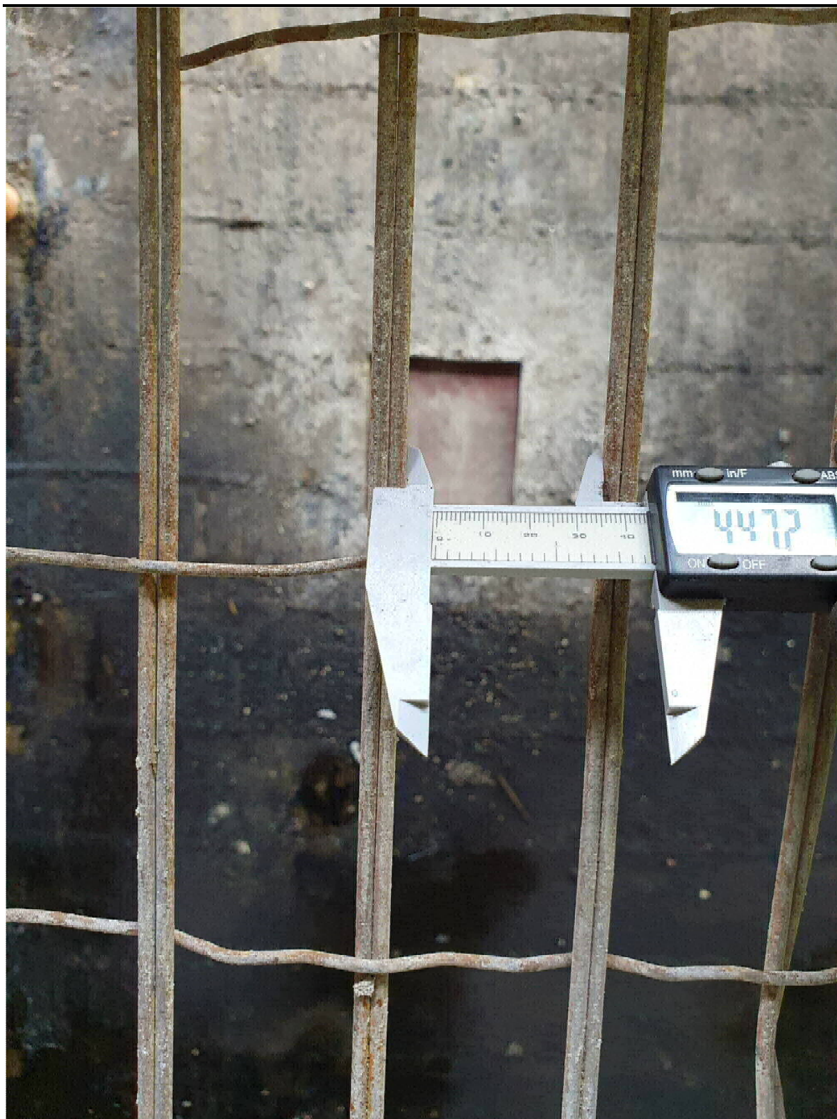
Slab Reinforcing Steel
