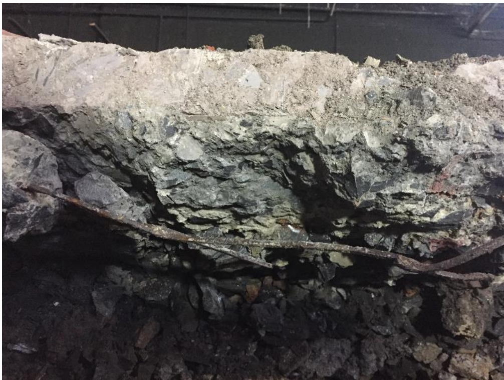
Photo 22: Ground Floor Slab
