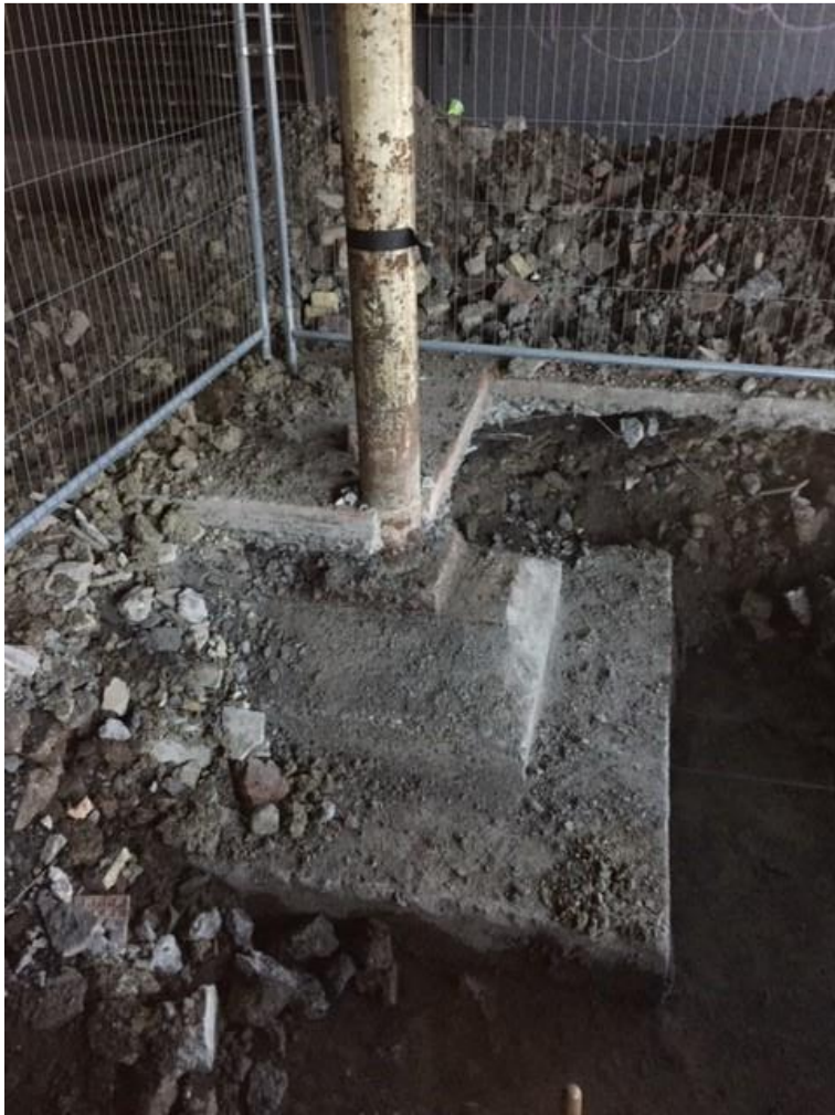
Photo 28: Tiered spread footing
