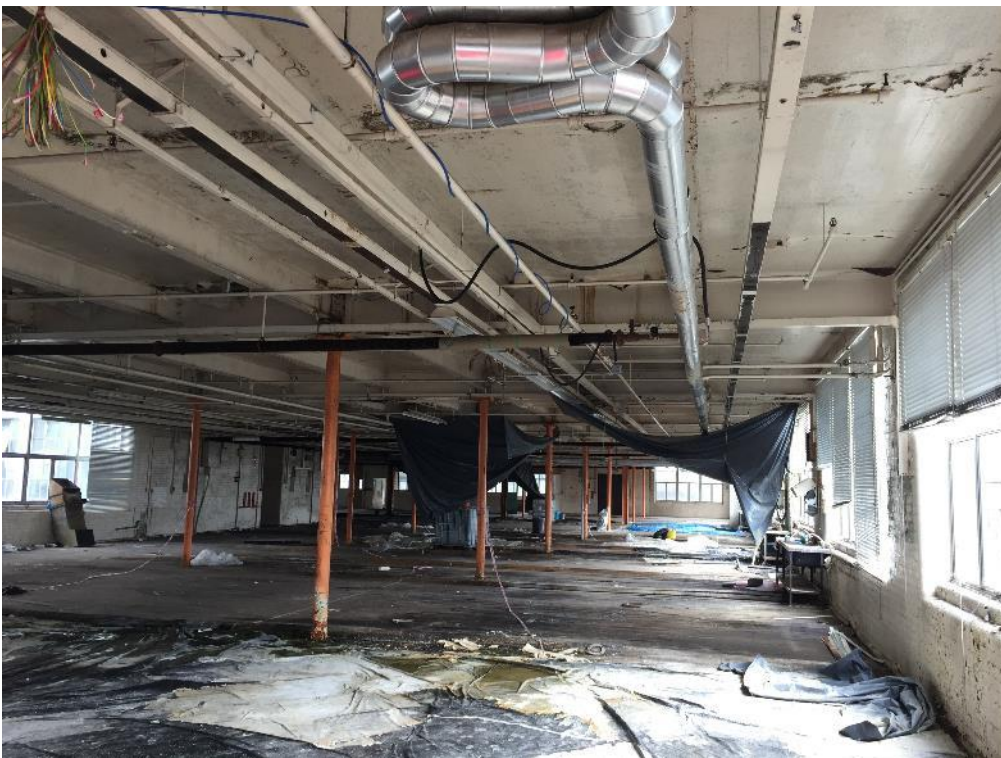
Photo 4: Original Building Condition
