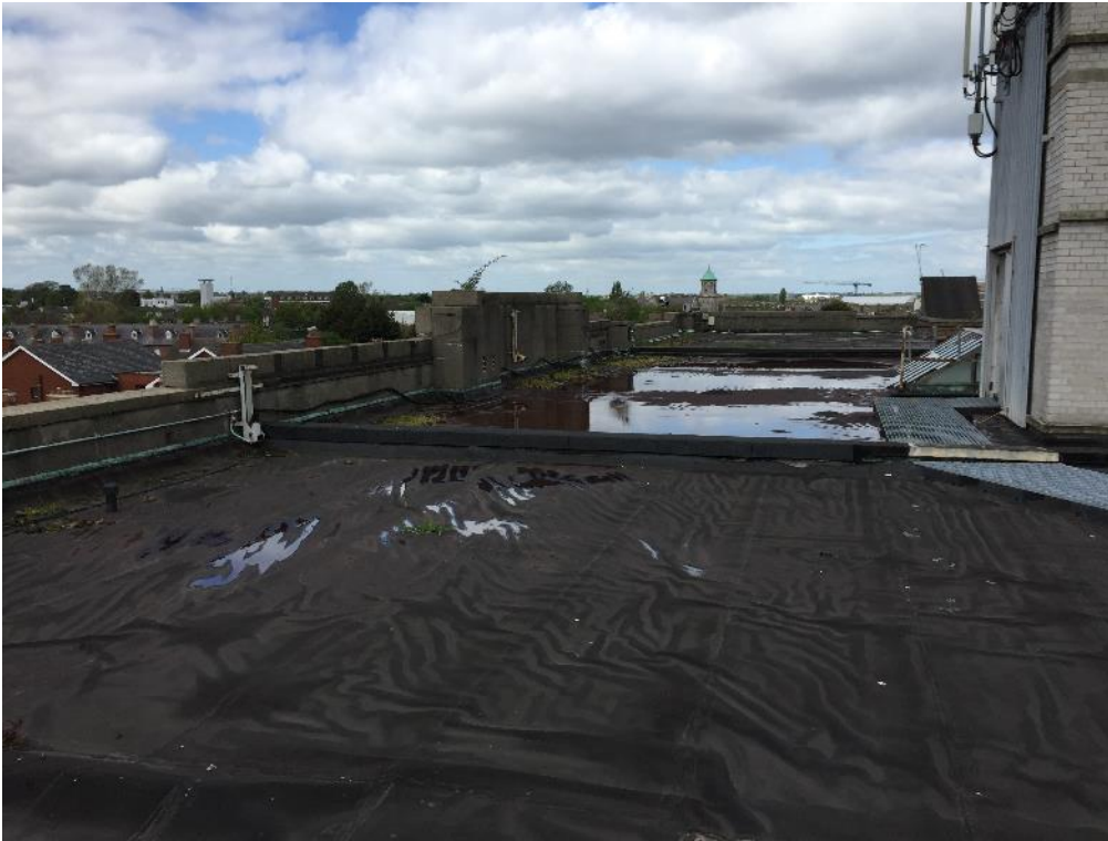
Photo 10: Original Building Condition
