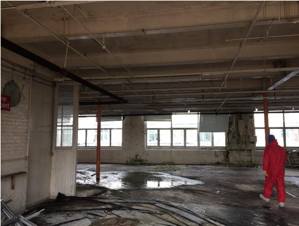
Photo 3: Original Building Condition
