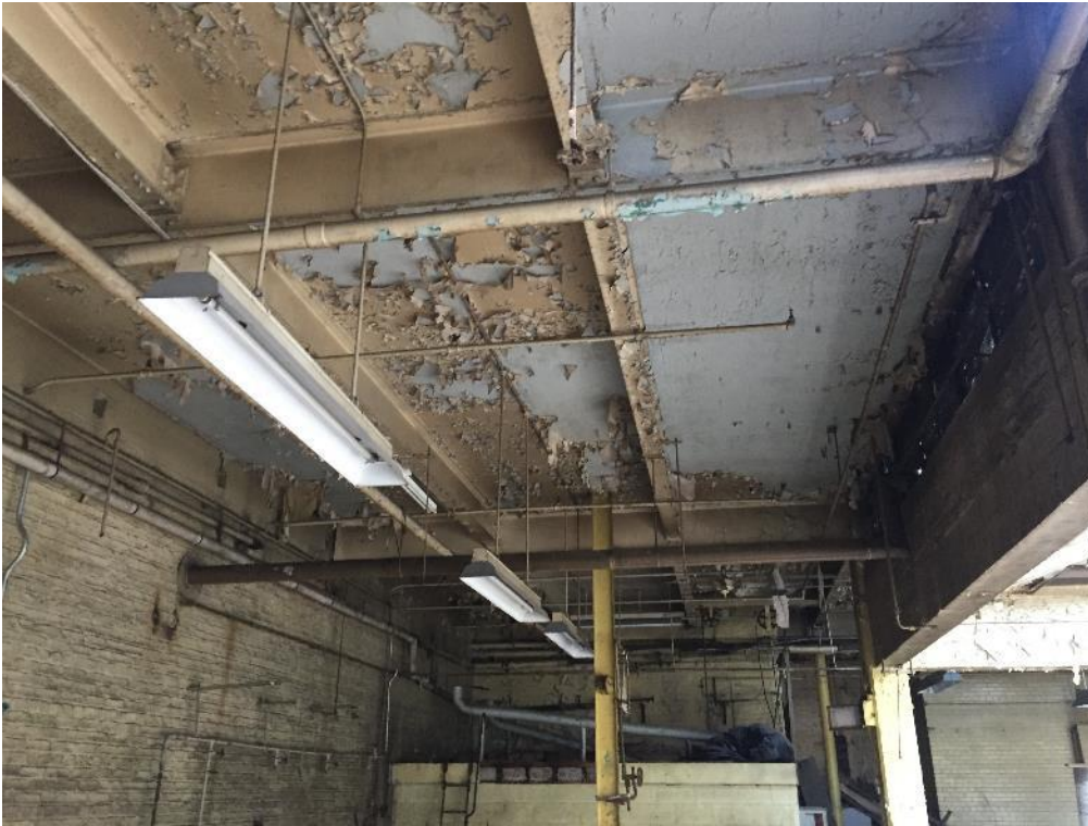
Photo 1: Original Building Condition
