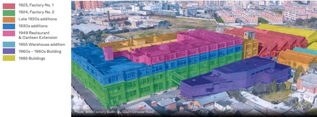
Figure 1.1 – Player Wills Factory – Construction Stages.
