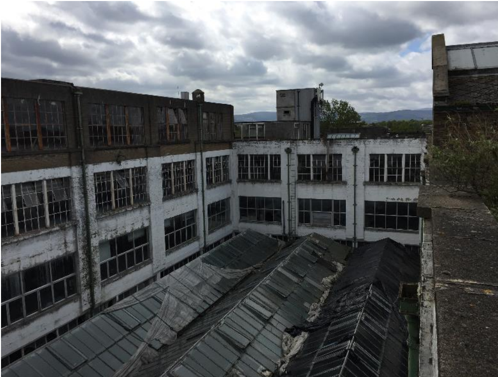
Photo 8: Original Building Condition
