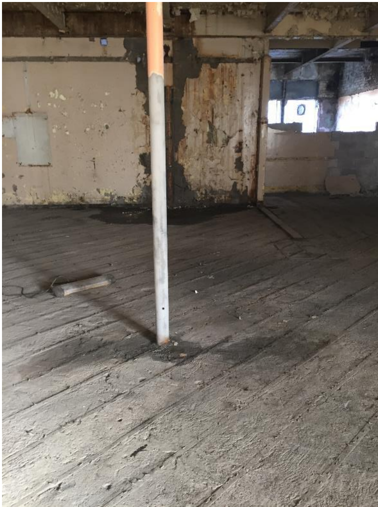
Photo 14: Level 2 column for 1920's section
