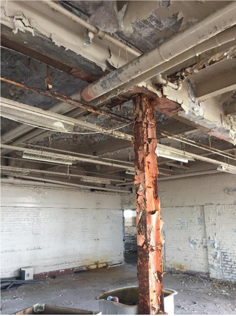
Photo 7: Original Building Condition
