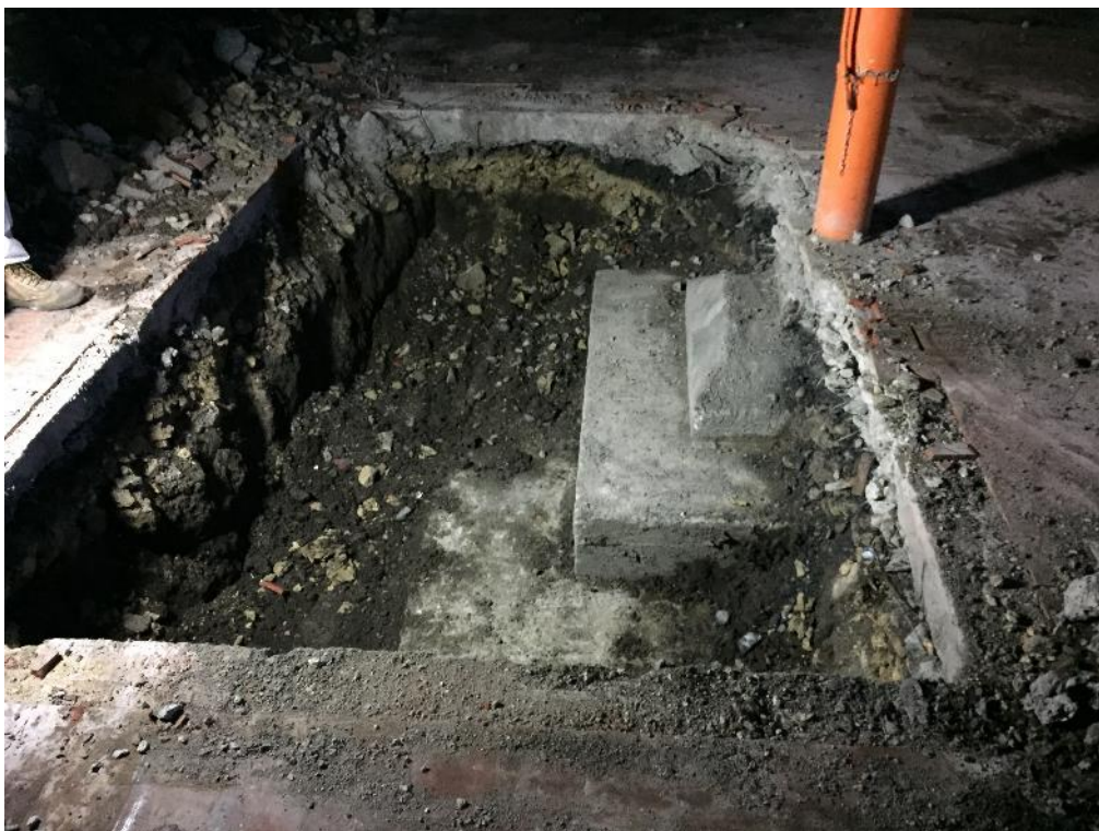
Photo 30: Tiered spread footing
